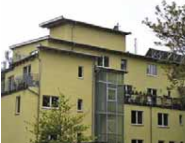
Multy family dwelling, 'Hohe Strasse', Hannover, Germany. Source: UCD Energy Research Group.
