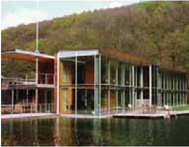
Passivhaus Eusenstadt, Austria. Source: Construct Ireland Issue 2, Vol 3.
