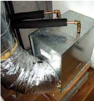
Water to air heat exchanger unit. Source: MosArt Architecture.
