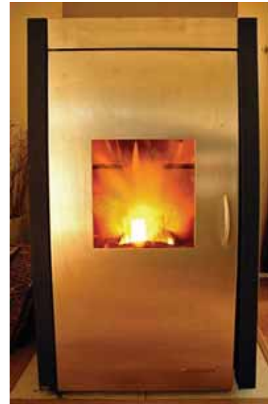
A pellet stove is at the hearth of an Irish passive house. Source: MosArt Architecture.
