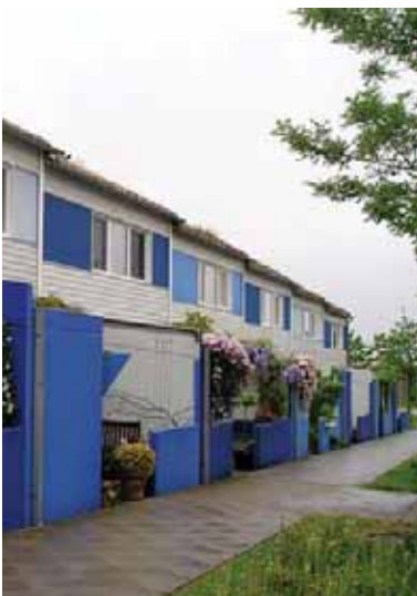
Kronsberg Passivhaus Complex Hannover, Germany. Source: UCD Energy Research Group.
