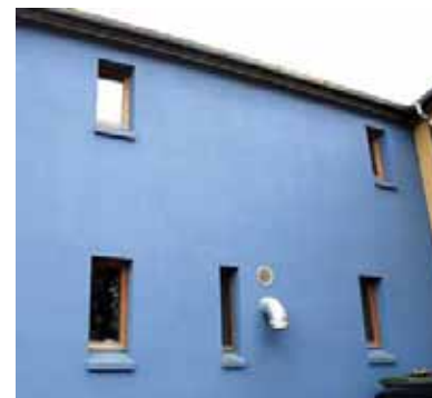
Windows on the northern elevation should ideally be small. Source: MosArt Architecture.
