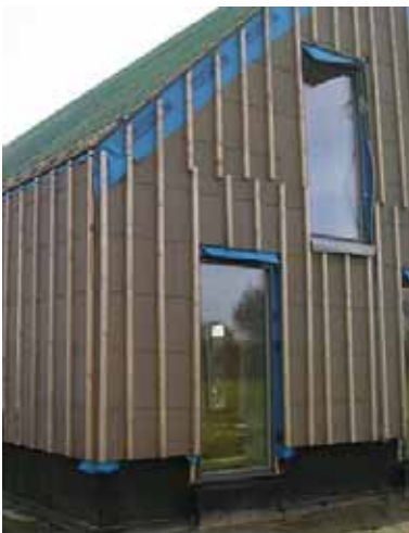
Timber frame house pre-cladding fitted airtight membrane. Source: Passivhaus Institut, Germany.
